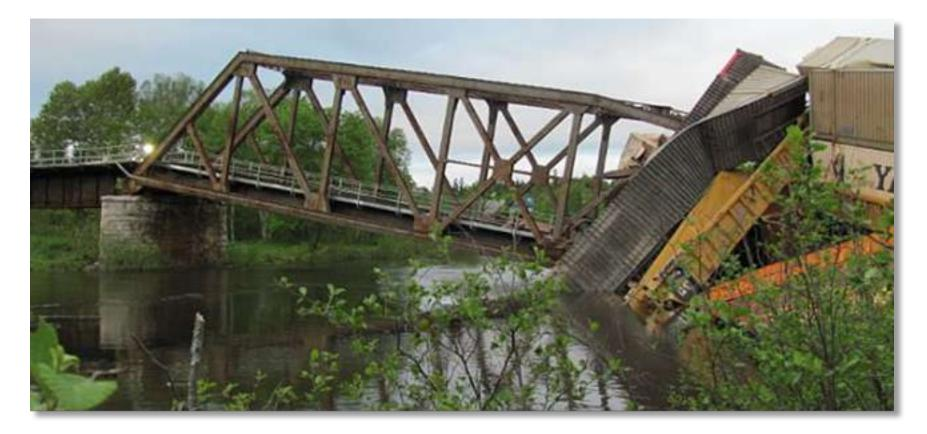
Wanapitei River, 2013: Wheel bearing failure sends 2 containers to river bottom and 5 floating
